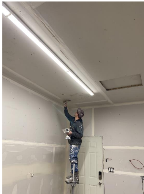
Figure 4: A worker mudding the ceiling while on stilts.
