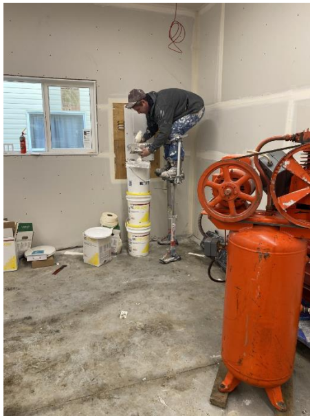
Figure 3: An example of a worker using stilts to mud the upper portions of a wall and ceiling. The pail of mud needed to be elevated for the worker to bend down to refill his pan with drywall mud.
