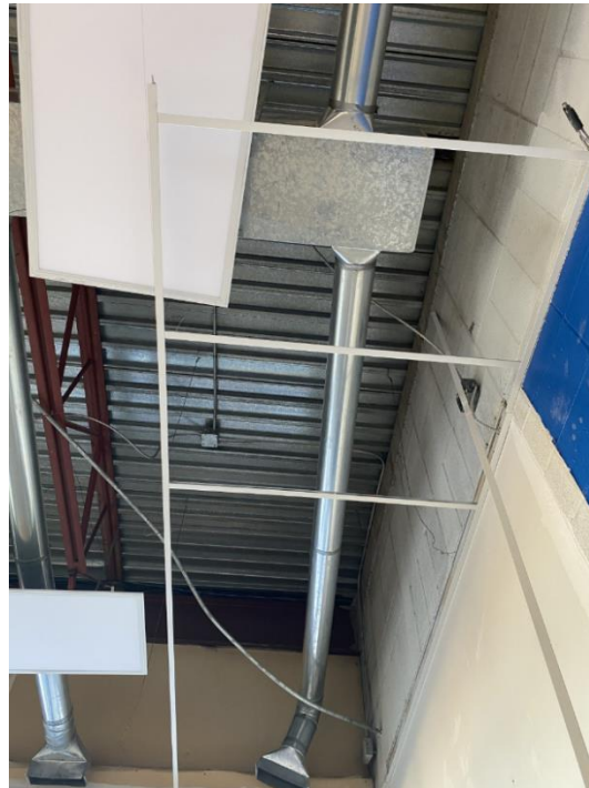
Figure 4: A section of the suspended ceiling that was completed. The Main T is running length wise, while the Cross Ts are running horizontally.
