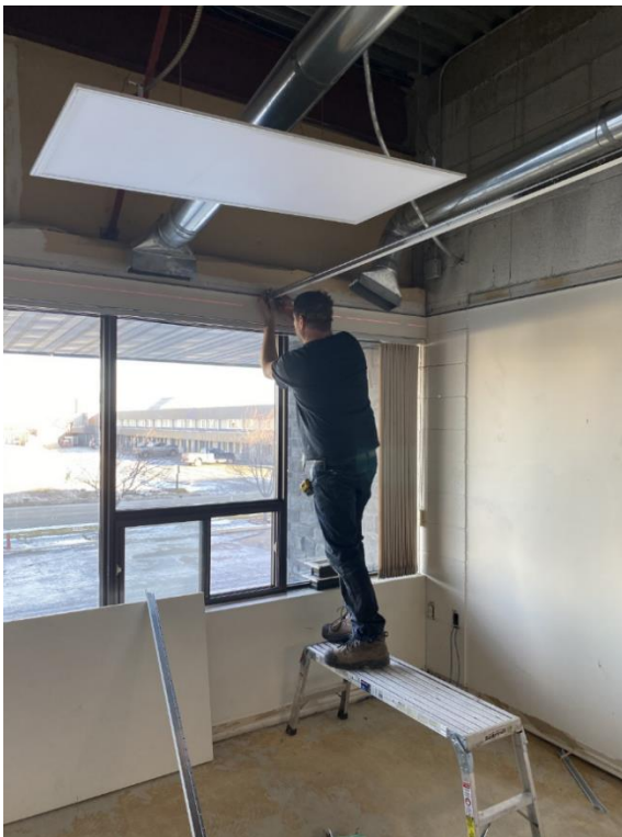
Figure 3: A worker installing a main T onto the wall and ensuring all angles are right.
