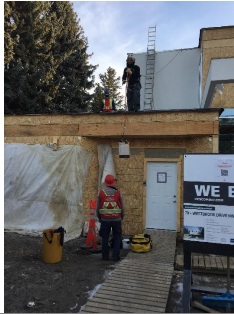
Figure 4: A Field Installer measuring flashing to ensure it will fit accurately on the corner of the parapet.
