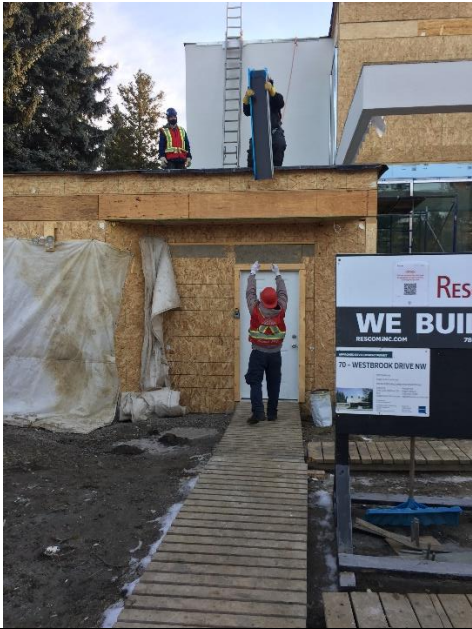
Figure 3: The worker transporting a pylon on the roof using the manual (rope) method.
