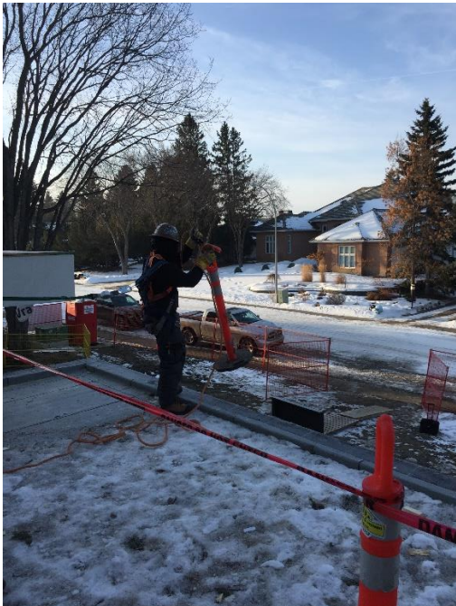
Figure 3: The worker transporting a pylon on the roof using the manual (rope) method.
