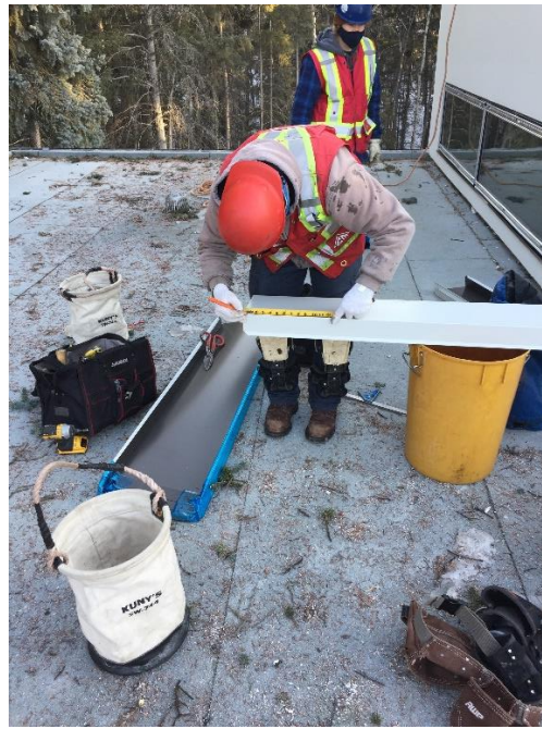
Figure 4: A Field Installer measuring flashing to ensure it will fit accurately on the corner of the parapet.
