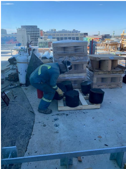
Figure 3: Roofer operating hi-boy in preparation to transport tar.
