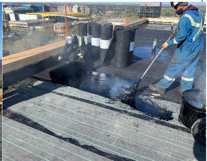
Figure 4: Using the tar mop in order to install felt membrane.
