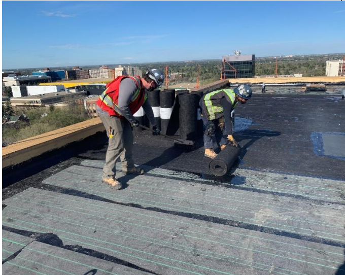
Figure 5: Securing the felt membrane by pushing/pulling a push broom.
