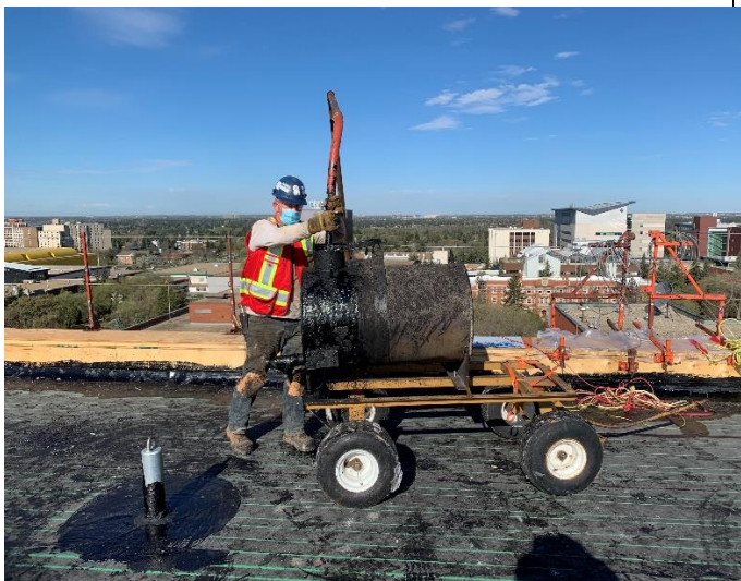
Figure 3: Roofer operating hi-boy in preparation to transport tar.
