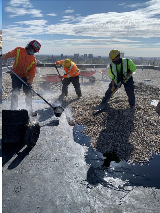
Figure 6: Securing the gravel to the membrane using a tar ladle and spades/shovels.
