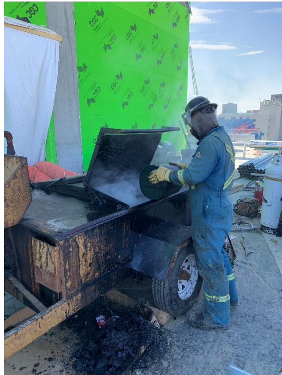
Figure 4: Using the tar mop in order to install felt membrane.
