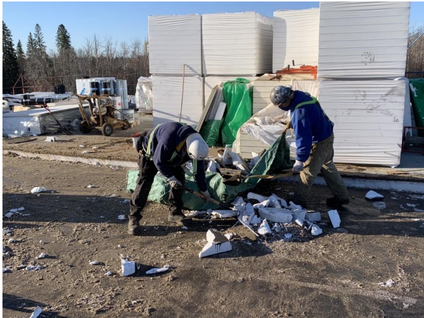
Figure 1: Using shovel to remove pre-existing material from roof during site clean up.
