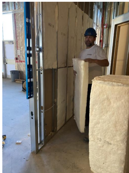
Figure 4: A worker placing the last insulation bat for the lower portion of the wall. The insulation is pictured to the right of the picture following the removal of the bag.
