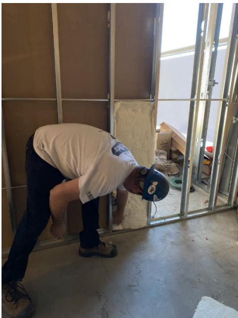
Figure 3: A worker insulating the lower portion of the wall.
