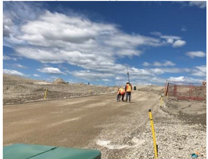
Figure 4: Using level to verify gradient
