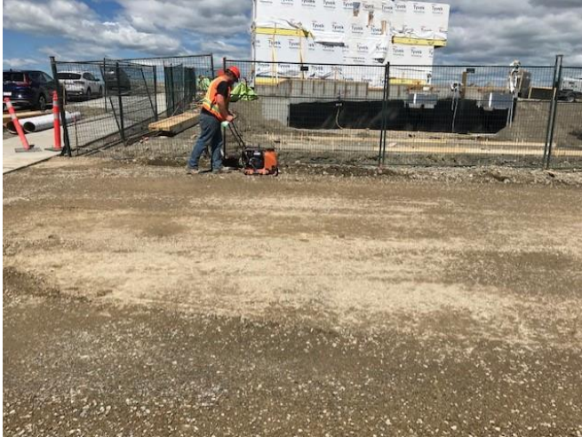
Figure 1: Using tamper to level out roadway
