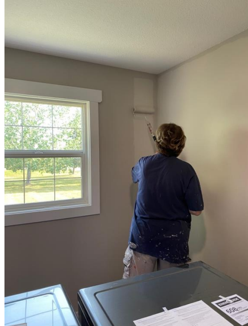
Figure 4: Pictured below is a worker rolling paint in a room that has already been cut.
