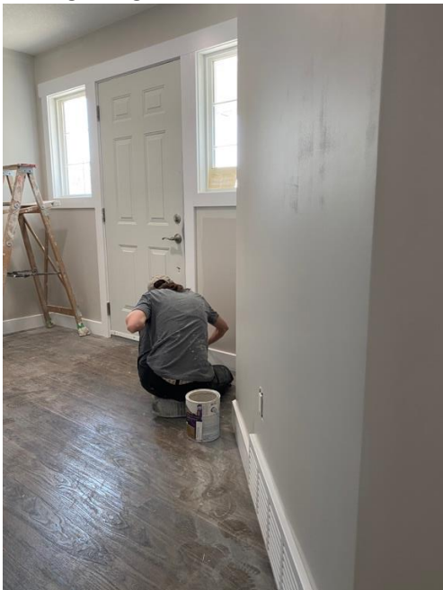
Figure 3: Pictured below is a worker completing cutting along the baseboards of a wall.
