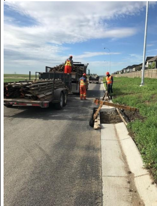
Figure 7: Unloading forms from truck bed, and forms placed in hole for use
