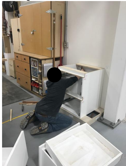
Figure 4: Securing lower cabinet to wall
