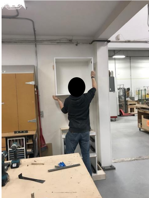
Figure 7: Placing upper cabinet on ledger
