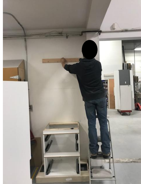
Figure 8: Securing upper cabinet to wall
