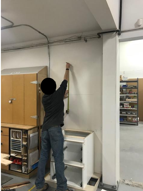
Figure 7: Placing upper cabinet on ledger
