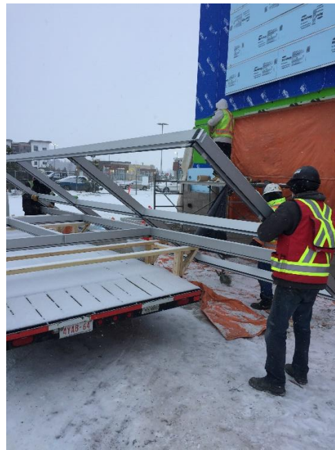
Figure 4: Using a shoulder carry method to carry the frame to the opening.
