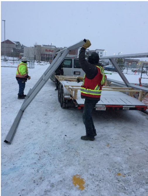
Figure 3: Holding the frame steady while a coworker adjusts the frame to lean onto the work trailer.
