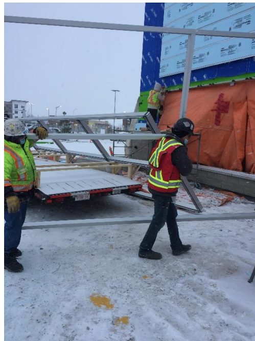
Figure 4: Using a shoulder carry method to carry the frame to the opening.
