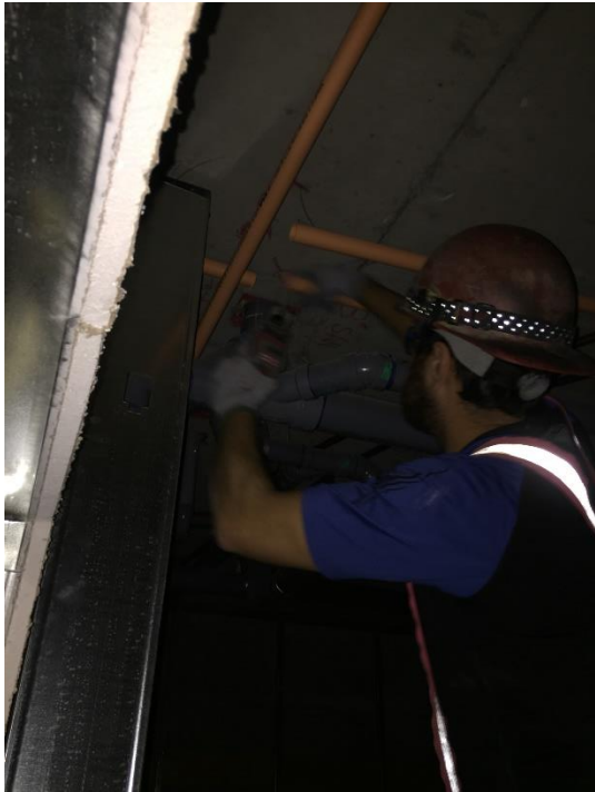
Figure 3: Sprinkler system installed under stair case.
