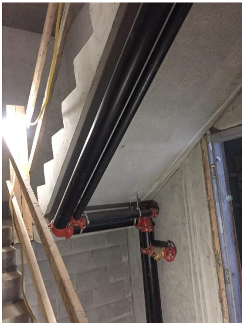
Figure 3: Sprinkler system installed under stair case.
