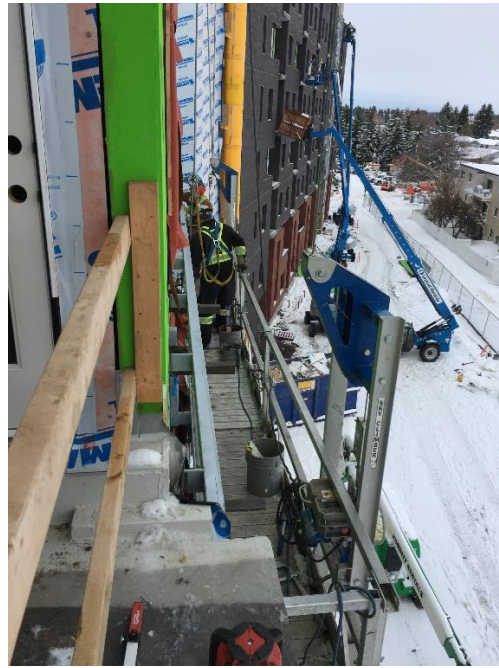
Figure 2: Ironworkers on swing stage working together to install brick angle.
