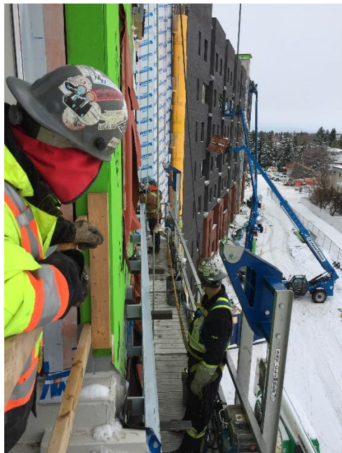
Figure 3: Ironworker observing as coworker installs brick angle using welding technique.
