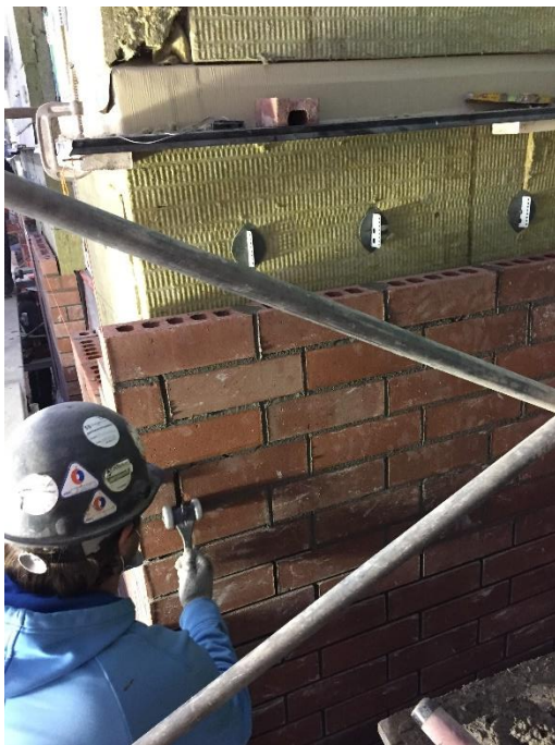
Figure 3: Kneeling while using raker to provide finished look to the bricks. Often completed every 100 bricks laid.
