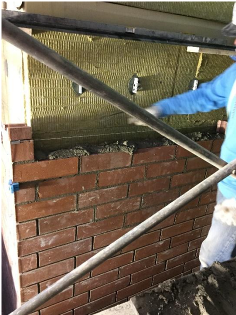
Figure 3: Kneeling while using raker to provide finished look to the bricks. Often completed every 100 bricks laid.
