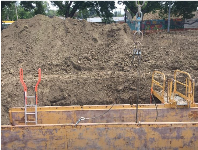
Figure 3: Direct view in trench box with pipe and pea gravel.
