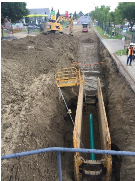
Figure 3: Direct view in trench box with pipe and pea gravel.
