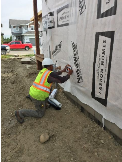
Figure 1: Measuring and installing plumbing to site exterior.
