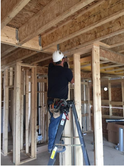
Figure 1: Using hole saw to install duct.
