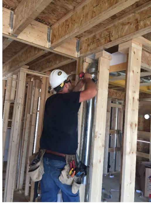
Figure 2: Drilling to install duct.
