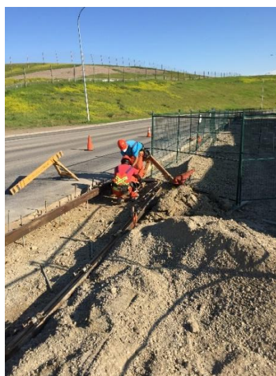
Figure 6: Cutting wooden slats at appropriate length to place in between wooden boards and concrete.
