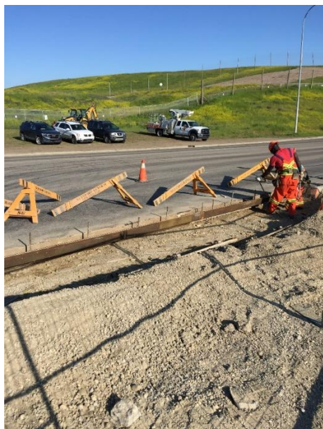
Figure 3: Hammering nails into wooden boards to secure in place.
