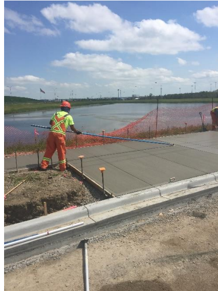
Figure 4: Concrete Finishers crouching and kneeling while using hand trowels.
