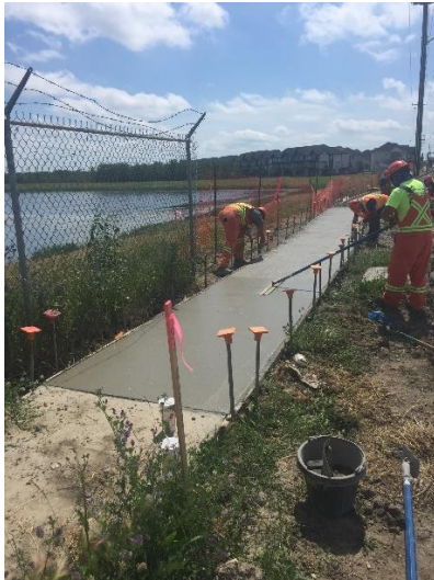
Figure 3: Concrete Finisher completing over shoulder reaching while using bow float.
