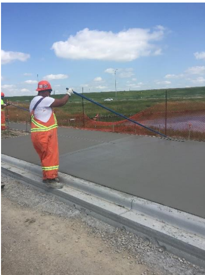
Figure 3: Concrete Finisher completing over shoulder reaching while using bow float.
