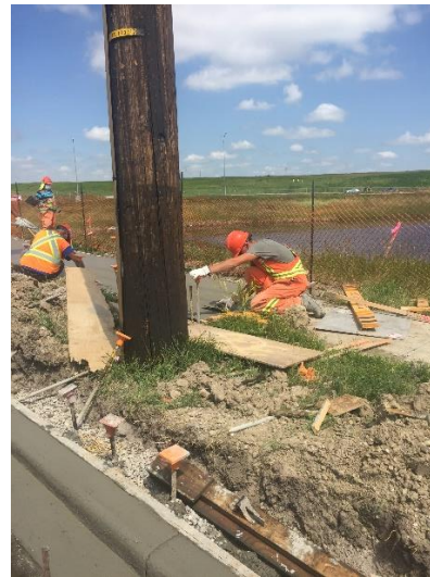
Figure 4: Concrete Finishers crouching and kneeling while using hand trowels.
