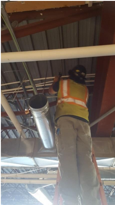
Figure 3: Overhead Water Line Work
