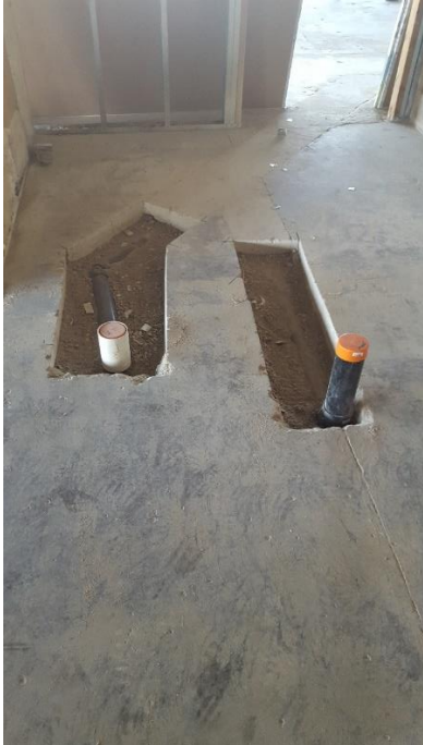
Figure 1: Ground work/Rough in
