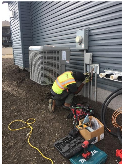
Figure 4: Installing power to air conditioning unit.
