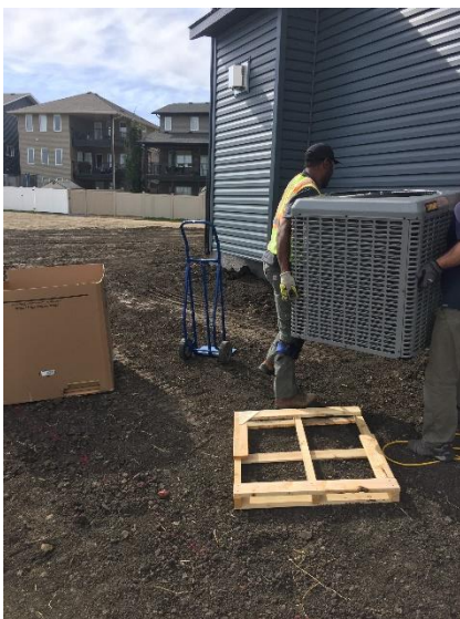
Figure 3: Lifting and carrying air conditioning unit onto bracket for installation.
